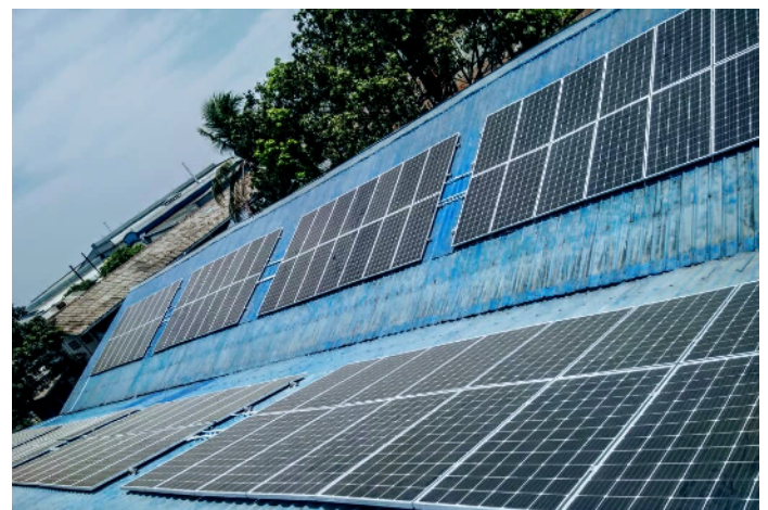
Shwe Zarmani, an SME garment factory in Yangon, installed a 66 kW solar PV system with Mandalay Yoma in early 2019.
