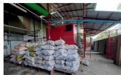
Well-Protected Fuel Storage Area
