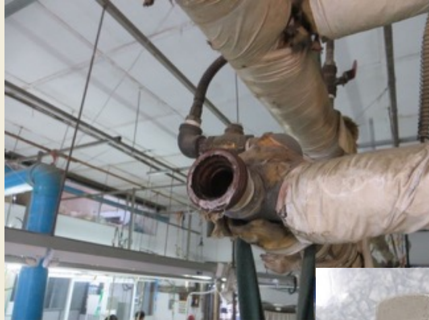
Operation of steam trap replacement at factory J
